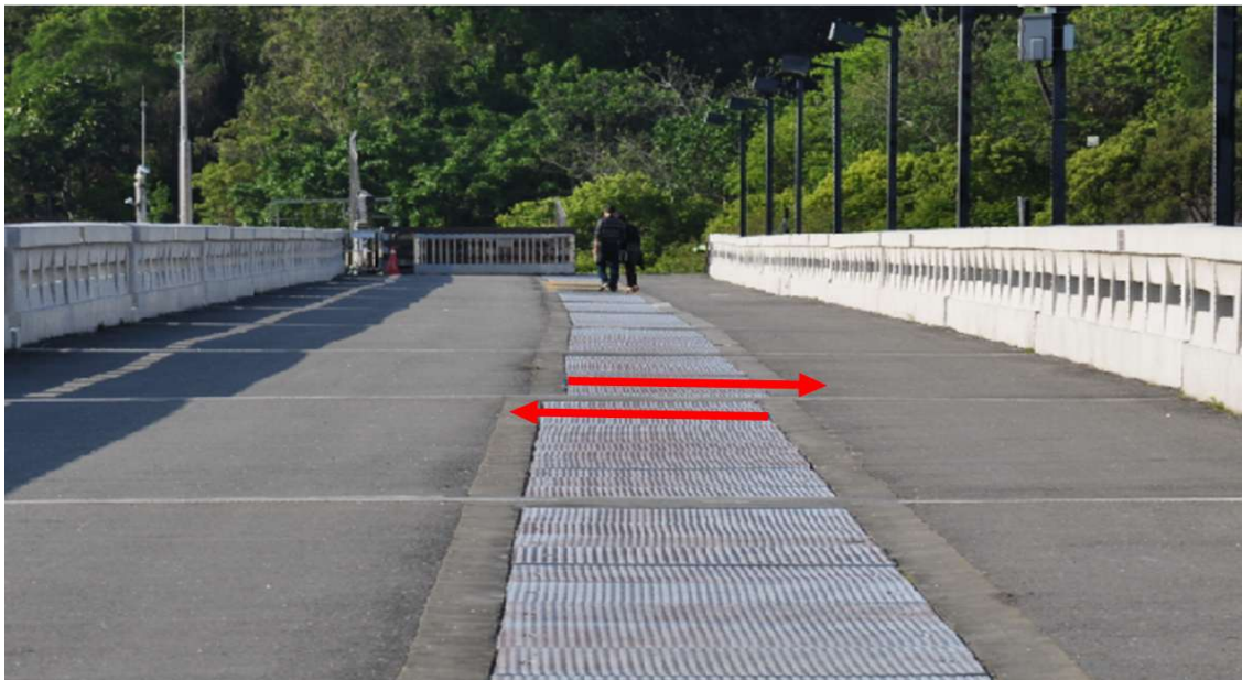
Figure 6. Horizontal shear banding observed at Shi-gang Dam
