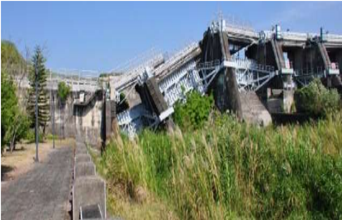
Figure 5. The shear banding triggered significant uplift, resulting in damage to the Shi-gang Dam.
